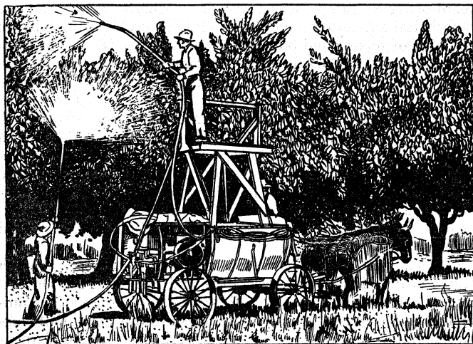
BY COURTESY OF U.S. DEPT. OF AGRICULTURE, BUREAU OF ENTOMOLOGY AND PLANT QUARANTINE FIG. 2. — ORCHARD SPRAYER WITH TOWER. USED FOR SPRAYING APPLE ORCHARDS FOR CODLING MOTH AND OTHER INSECTS
